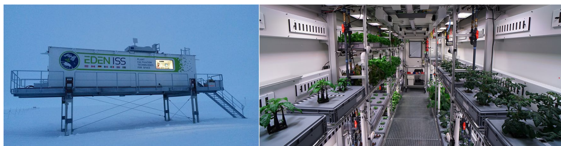
Fig. 2 An outside view of the MTF on its platform in Antarctica (left) and the FEG inside shortly after seeding (right). The interior holds grey boxes, which keep the plants in place and cover the aeroponic nutrient delivery system
